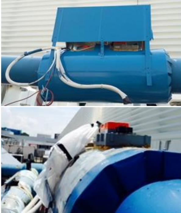
*Figure 5: Belimo Energy Valve™ installed on the SPMS building rooftop*
